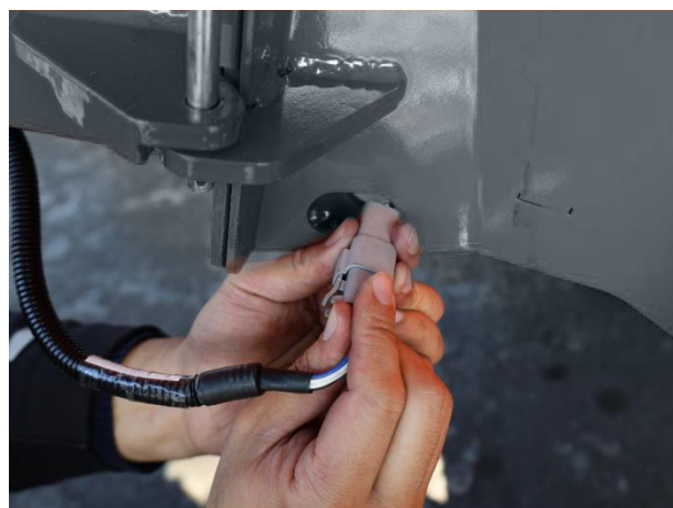
Control harness connection #2
